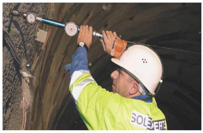
Figure 2.26 shows the installation of distometer in tunnel.
