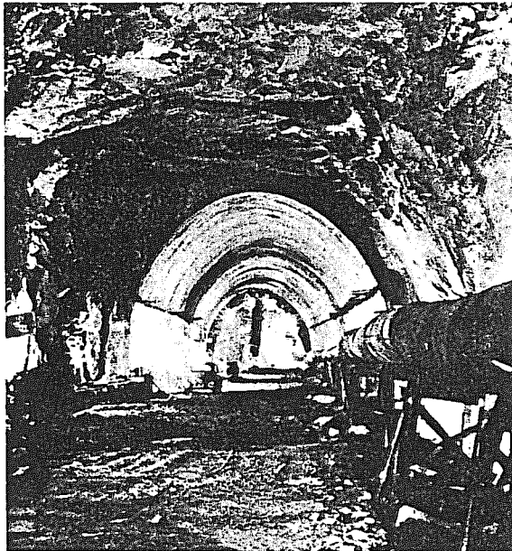
Figure 9 Two different blasting techniques applied in the same rock at the construction of adjacent roadway tunnels
