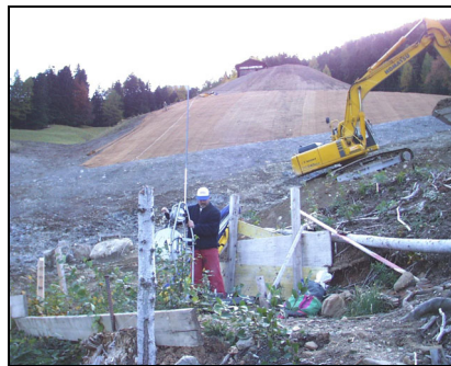
Fig. 3 New shape of the slope with coconut geo-mesh. After /2/ Frodl.
