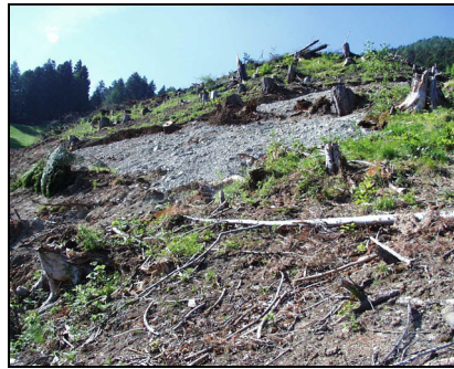
Fig. 2 Slope prior to excavation, May 2001. After /2/ Frodl.
