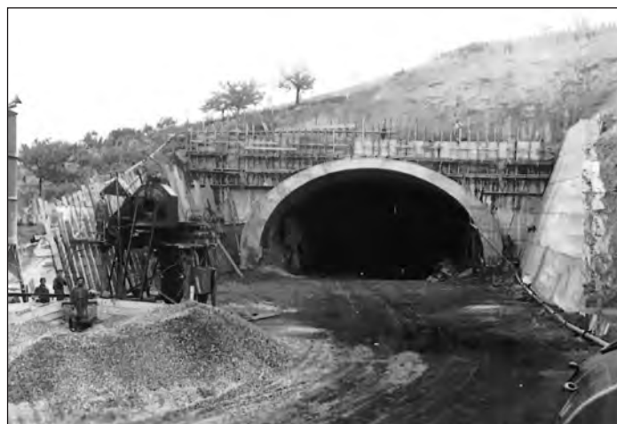
Le tunnel de Rive-de-Gier en construction / The Rive-de-Gier tunnel during construction.
